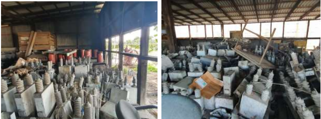
Oil Capacitors (non-PCB oil)
